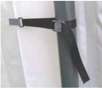
Pocket for side wall conduit
