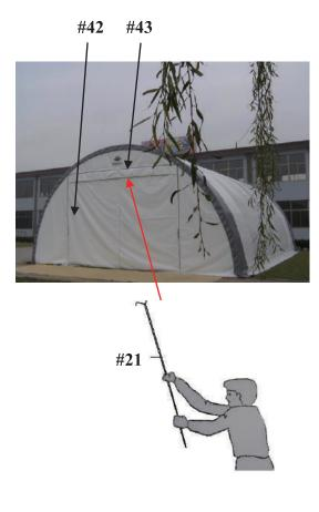
(in order to protect the shelter from heavy wind, please install the wind bracing straps at points 300 mm measuring from the ends, and others to be installed in the middle averagely.) (photos are for reference only, the real quantity is according to packing list.)
